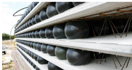
Fig 1.1:Bubble deck slab
