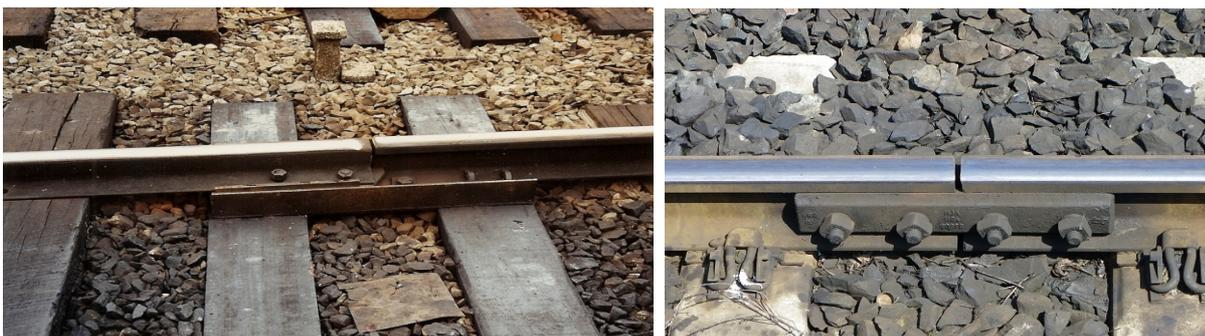
Fig: Tracks Connected By Nuts & Bolts
