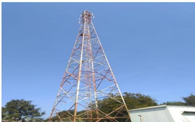
Fig.1 Ground Base Cellular Tower
