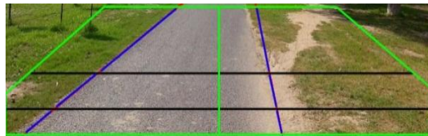
Fig 4 Detected road edges in different parts of ROI
