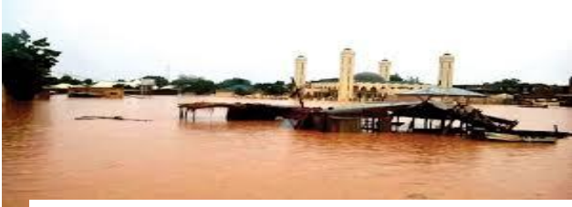
Fig 3 Flooded Rafin Atiku area
