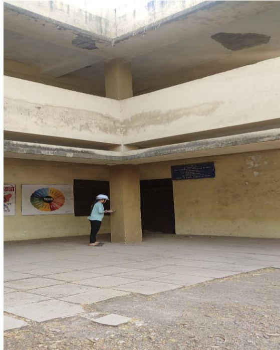
Fig.3 Column at Ground Floor
