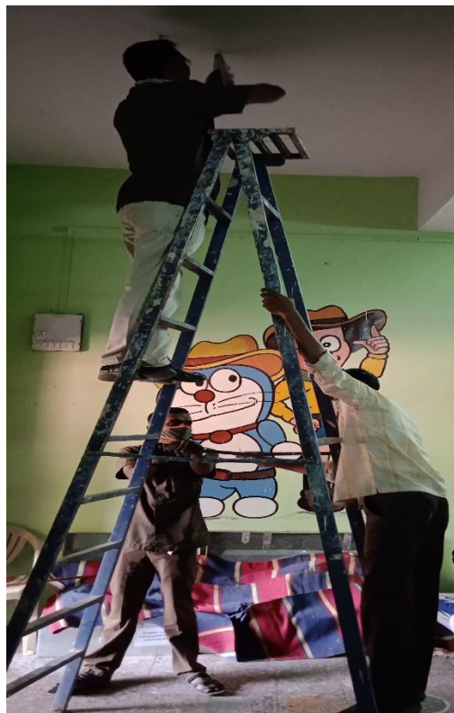
Fig.4 Slab of Class Room at Ground Floor
