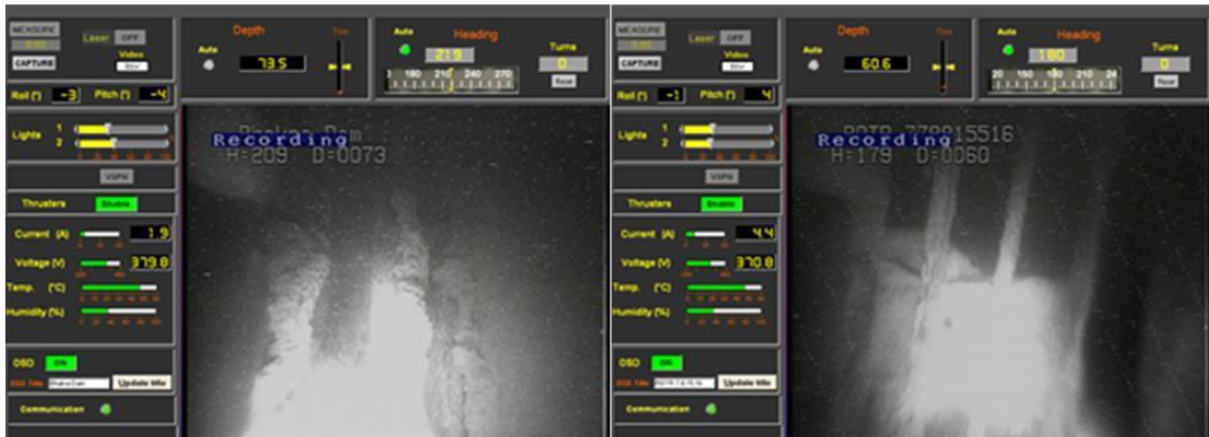
Trash rack of river outlet at 73 m depth Trash rack of river outlets at 60 m depth
