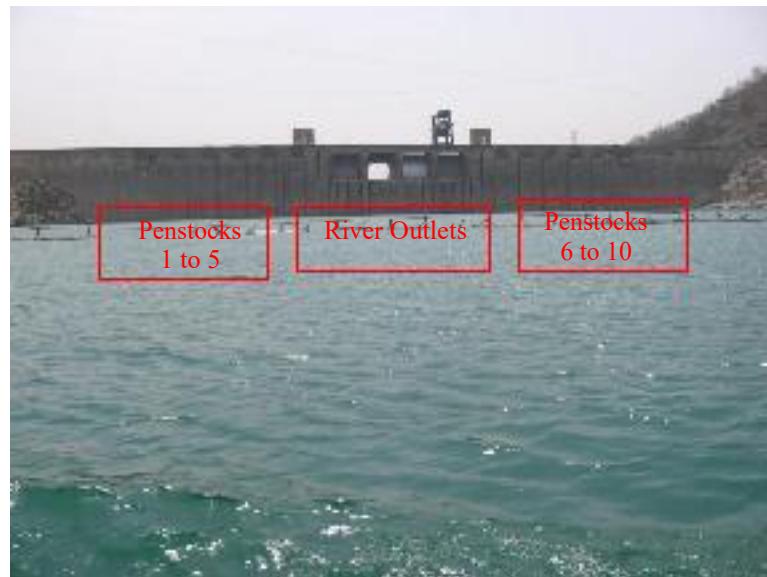
Fig. 1. Upstream face of Bhakra dam marked with penstocks and river
