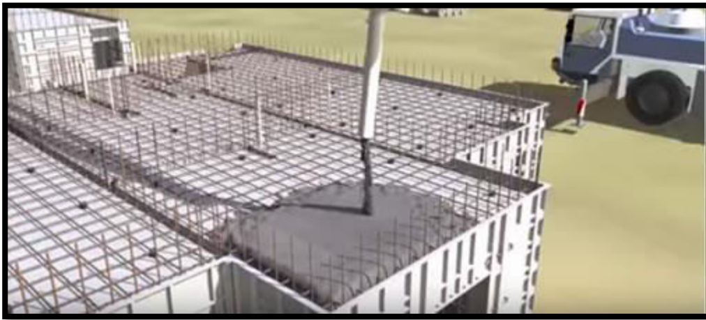
(Fig1.1 Monolithic Structure With Aluminum Formwork)
