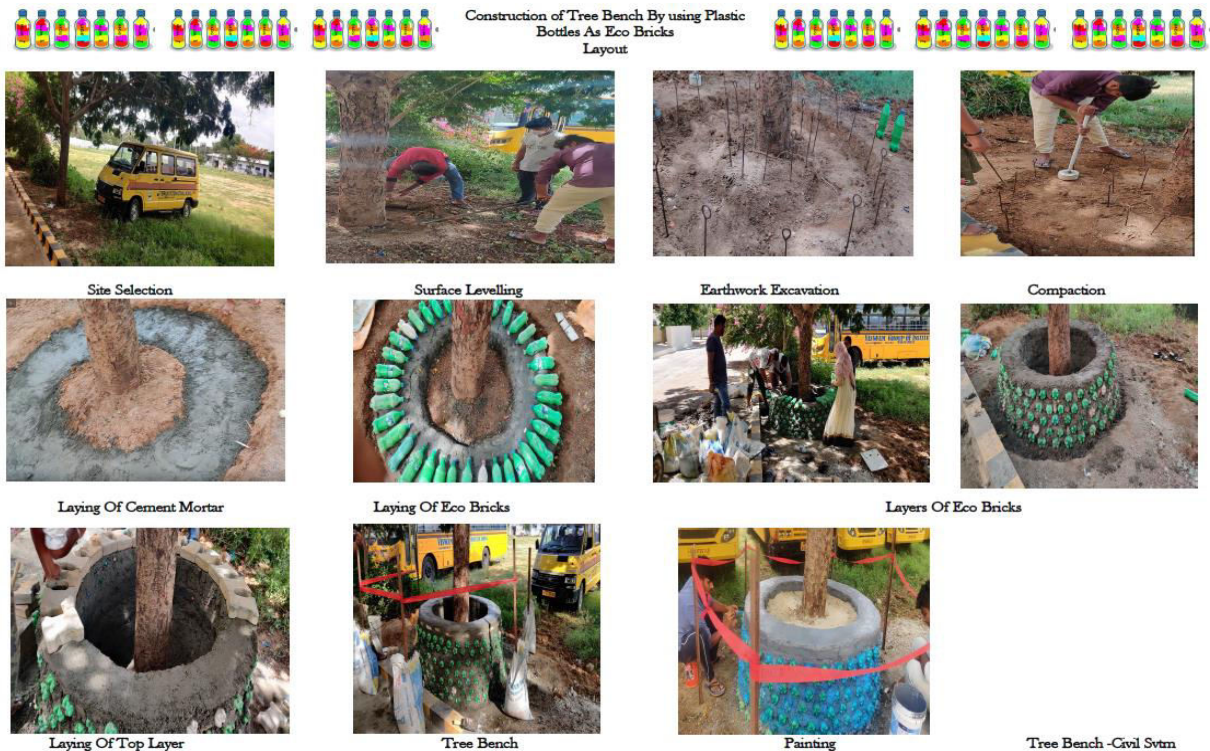
k. Tree Bench Construction
