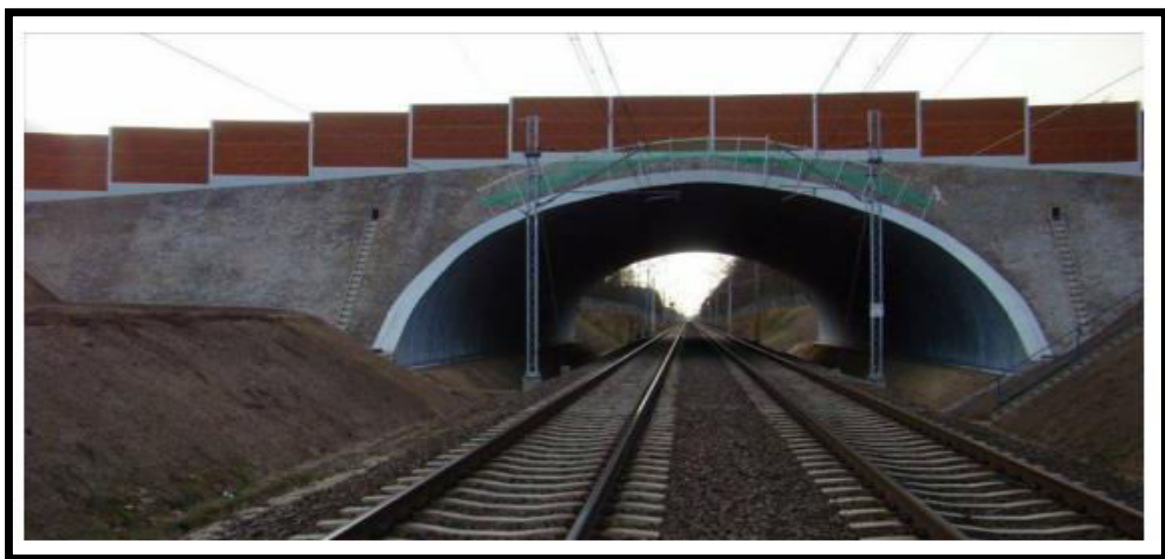
(Figure 2.2 By completing the steel structure with well-designed details, nice looking bridges can be achieved. This bridge is one of the largest SSCB in Europe having a 20 m span.)
