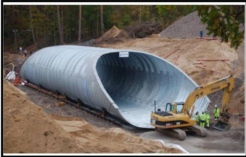
(Figure 2.1 The finalized erection of the steel part of a SuperCor horizontal ellipse bridge)
