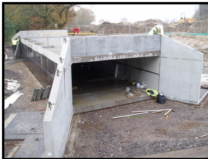
(Fig.1.1: RCC BOX CULVERT)
