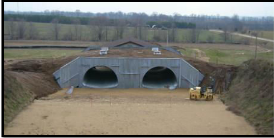
(Fig.1.2 :Pipe arch culvert. Source: http://www.theconstructor.org )
