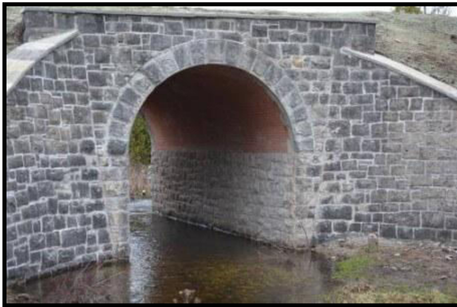
(Fig.1.4 :Arch culvert. Source: http://www.visitgrey.ca )
