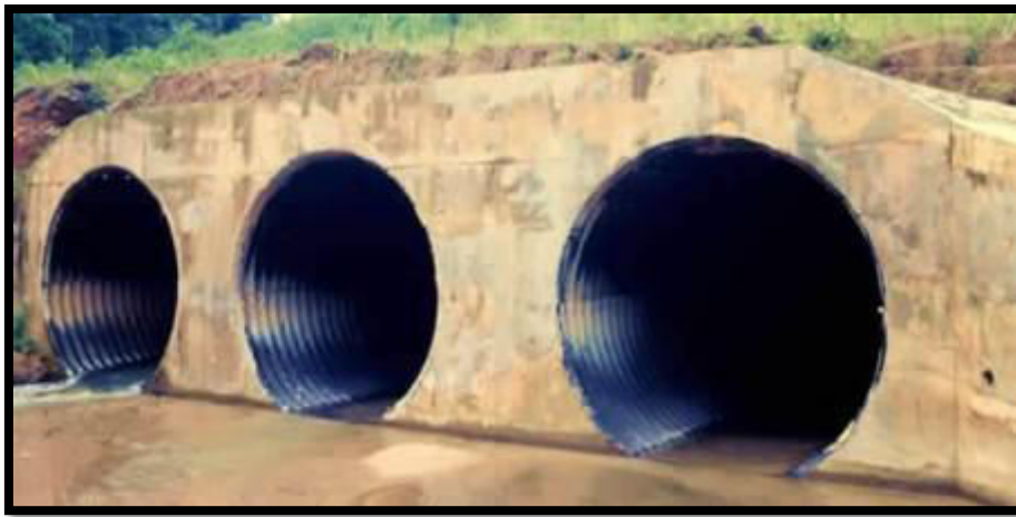
(Fig.1.1:Pipe culvert. Source: metal-culvert.com)
