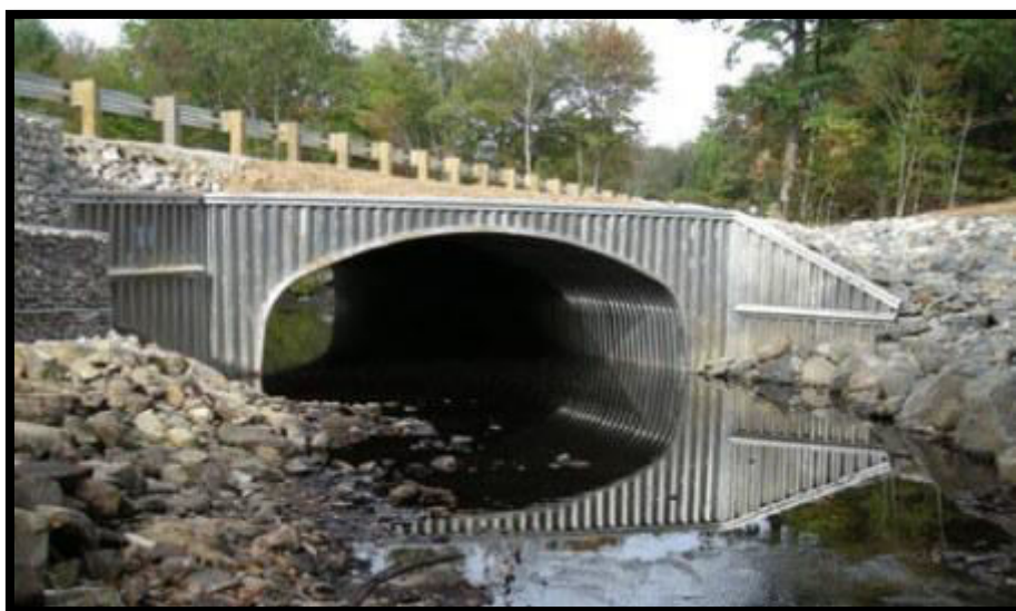
(Fig.1.6 :Metal Box Culvert. Source: conteches.com)
