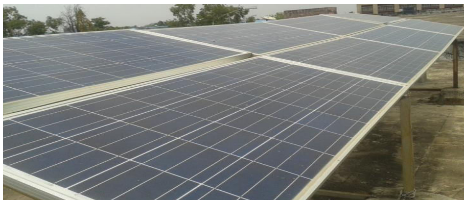
Figure 2: Solar Panel Installation
