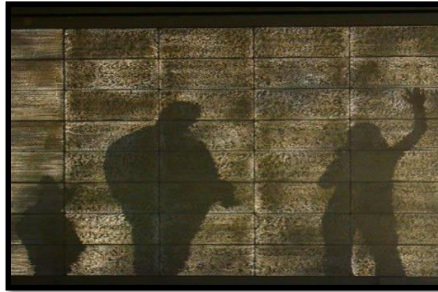
(Fig 5.2: Day view of litracon door from inside)
