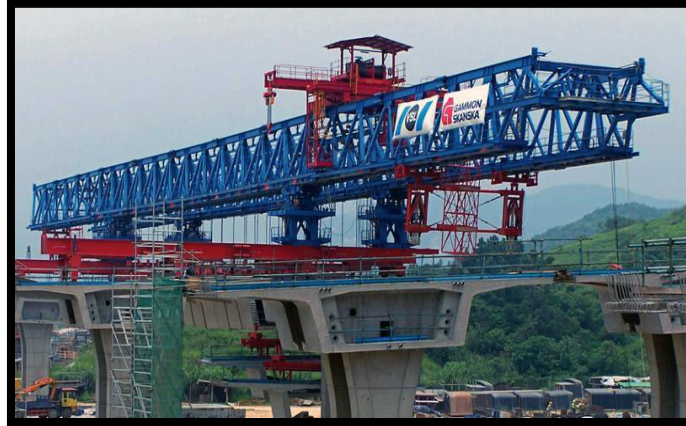
(Fig.1.4 : Construction of the girders using a launching truss)
