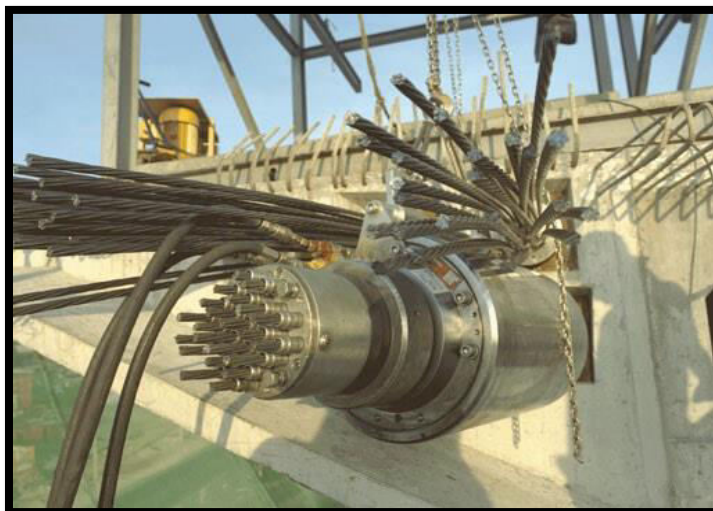
(Fig.1.6 : Post-tensioning of a bundle with strands)
