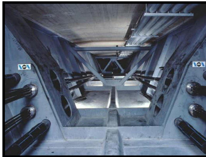
(Fig.1.5 : External prestressing tendons in the box girders)
