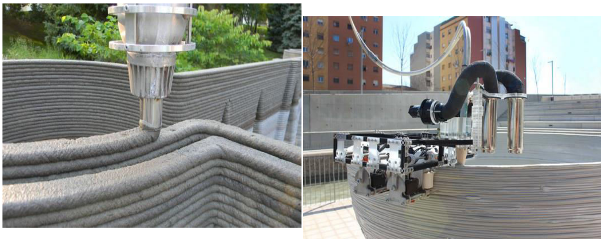
Fig 22: Robotic Arm Extruder
