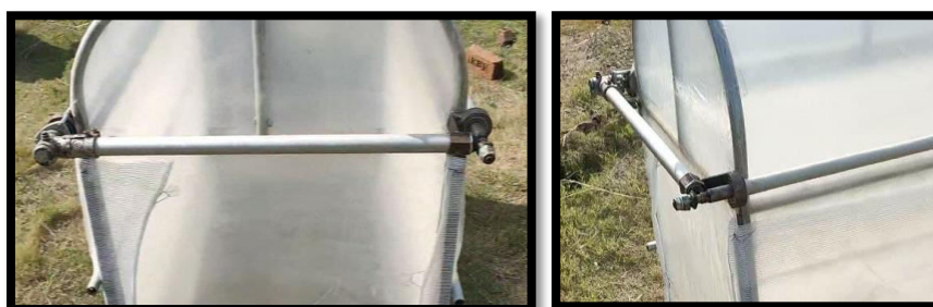
Fig 3: View of curtain operating mechanism
