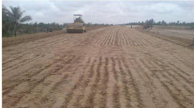
**Figure 1** Showing cement stabilised subgrade at test site
