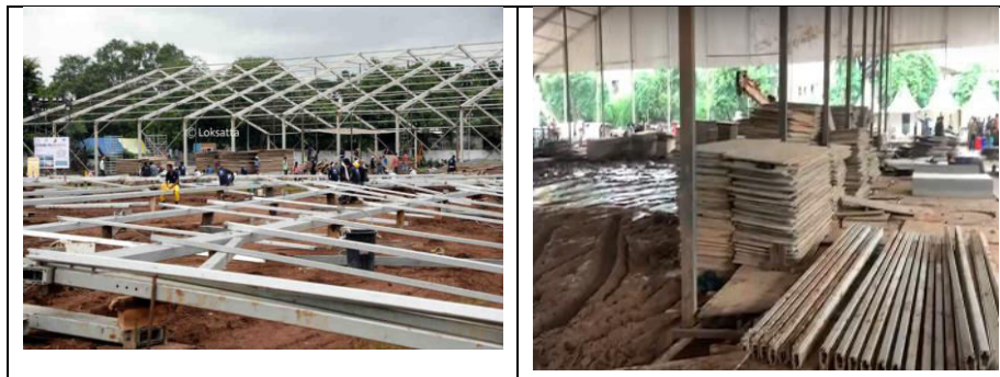
Fig.3: steel framing
