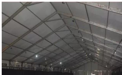
Fig.4: steel truss
