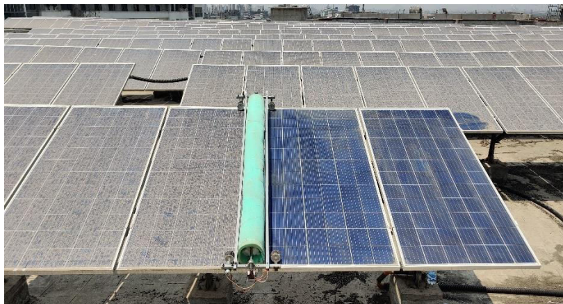
FIG. 3 Show Before and After Condition Of Solar Panel after Cleaning
