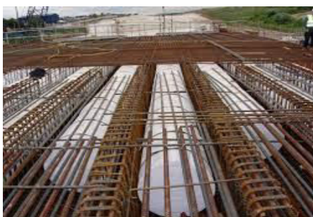
Fig.1. Voided deck slab
