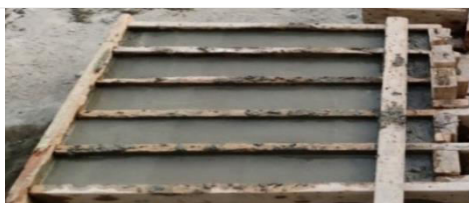
Fig 3: After Fibers Mixed With Concrete Placed in the Moulds
