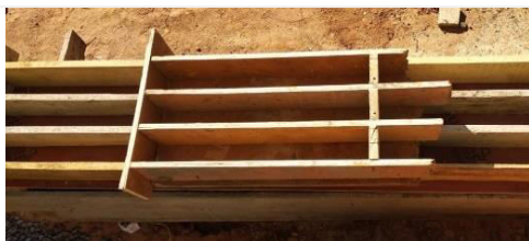
Fig.1: Preparation of Moulds
