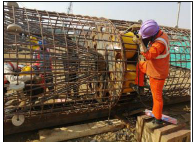
Installation process of O-Cell in cage
