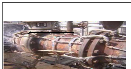
Figure 1: Steam Tracing Along Pipe Line (Wermac,2012)
