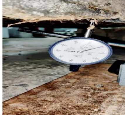
Figure 2 Strain gauge used for record the deflection
