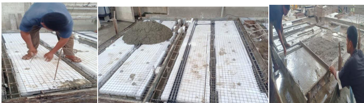
Fig. 3. Casting stages of precast walls using thermocole
