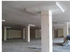
Fig.1.4 Flat slabs with Column Drop
