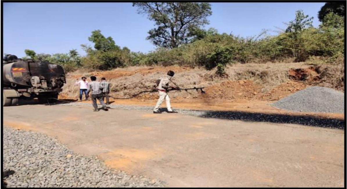
Figure No.3 Bitumen spray
