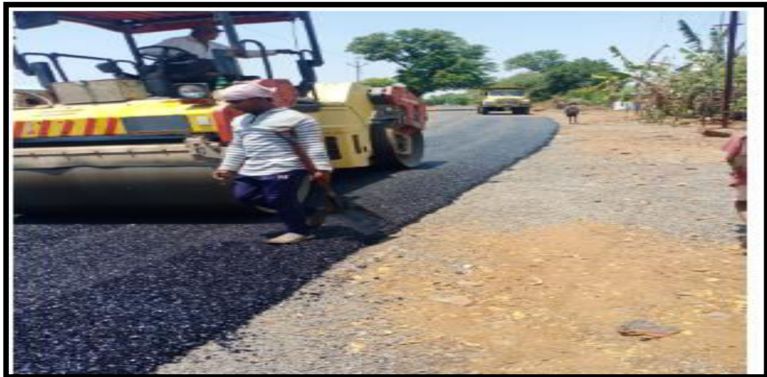
Figure No.4 Road compaction with the help of road roller
