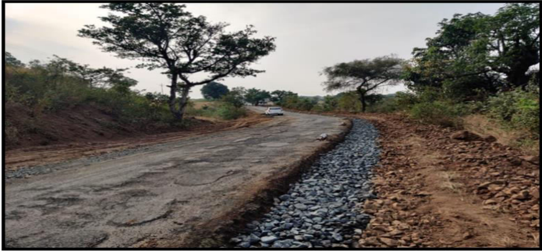
Figure No.5 Road Site
