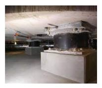
**E).** Base Separation: One of the ways to safeguard a structure against earthquakes is to use base isolation. It is a set of structural features designed to disconnect a superstructure from its substructure while it is lying on shaky ground, therefore safeguarding a building or non-building structure.
