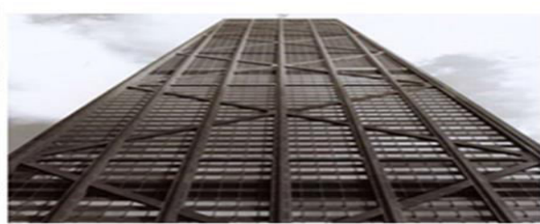
Fig 4: Cross bracing in building
