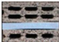
Fig.5 Composite wall with insulation
