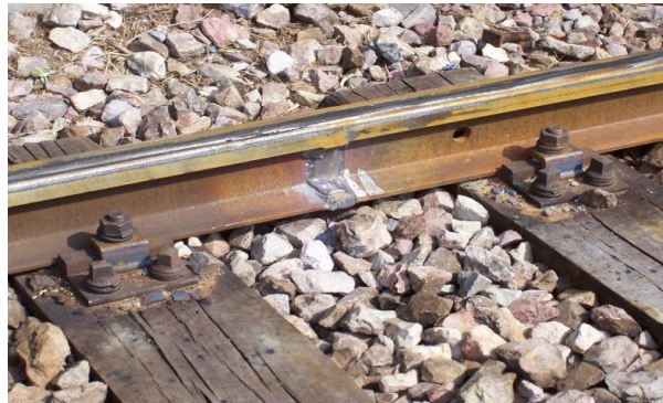
Fig1: Continuous welded rail
