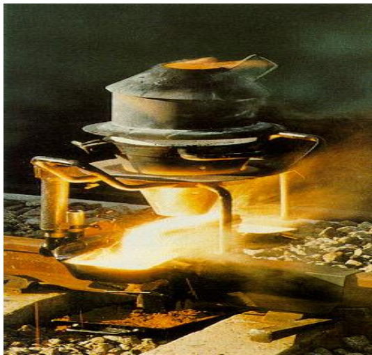
Fig 2: Thermite welding furnace
